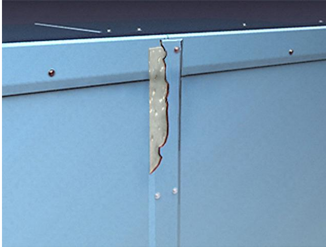
Figure 10: Joining Strip Detail.
